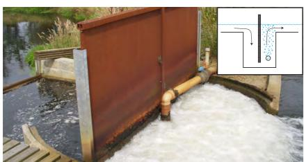
Figure 2.10 Aeration well system using the air-lift principle
