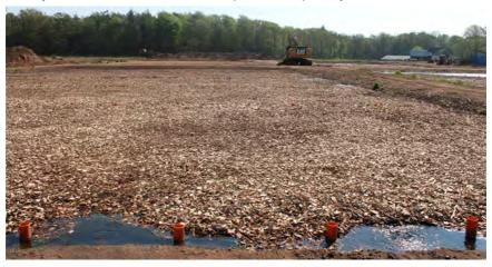
The filter shown holds 6 000 m³ woodchip for cleaning 100 L/sec reject water. The woodchip will acts as a carbon source for the denitrifying bacteria transforming nitrate into free nitrogen in an anaerobic environment.
