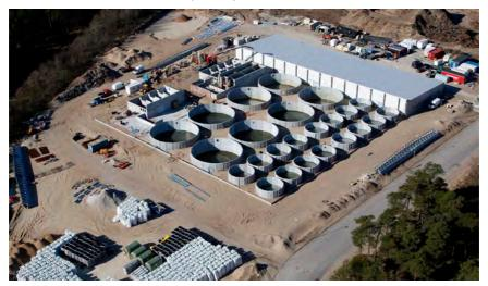
This 2 000 tonnes salmon farm in Hirtshals, Denmark was built in 2013. The system is based on recirculation technology and is covered by a building to control temperature and for high biosecurity. Salmon are grown from eggs to around 4–5 kg size in 2 years in large tanks of almost 1 000 m³ each. The white bigbags in the foreground are packed with biomedia ready to be filled into the biofilter chambers. Source: Axel Søgaard/AKVA group.
